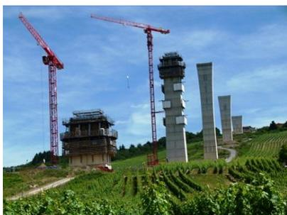
The two WOLFF cranes are being used for eight bridge pylons, the highest of which is 160 meters high. Several relocations of the cranes, including climbing and tie-ins make the project in the Mosel Valley, which is susceptible for winds, particularly challenging.
